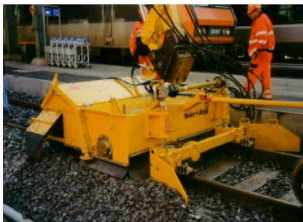
A rotating broom sweeps and feeds excess ballast onto a lateral conveyor belt for transport to either left or right side of the tracks as selected. All control functions are initiated from the driver's cabin of the excavator.
